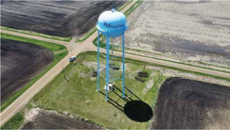
Aerial view of TM Rural Water tower
