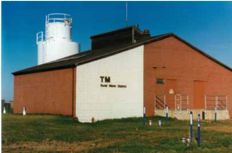
Original TM Water Treatment Plant
